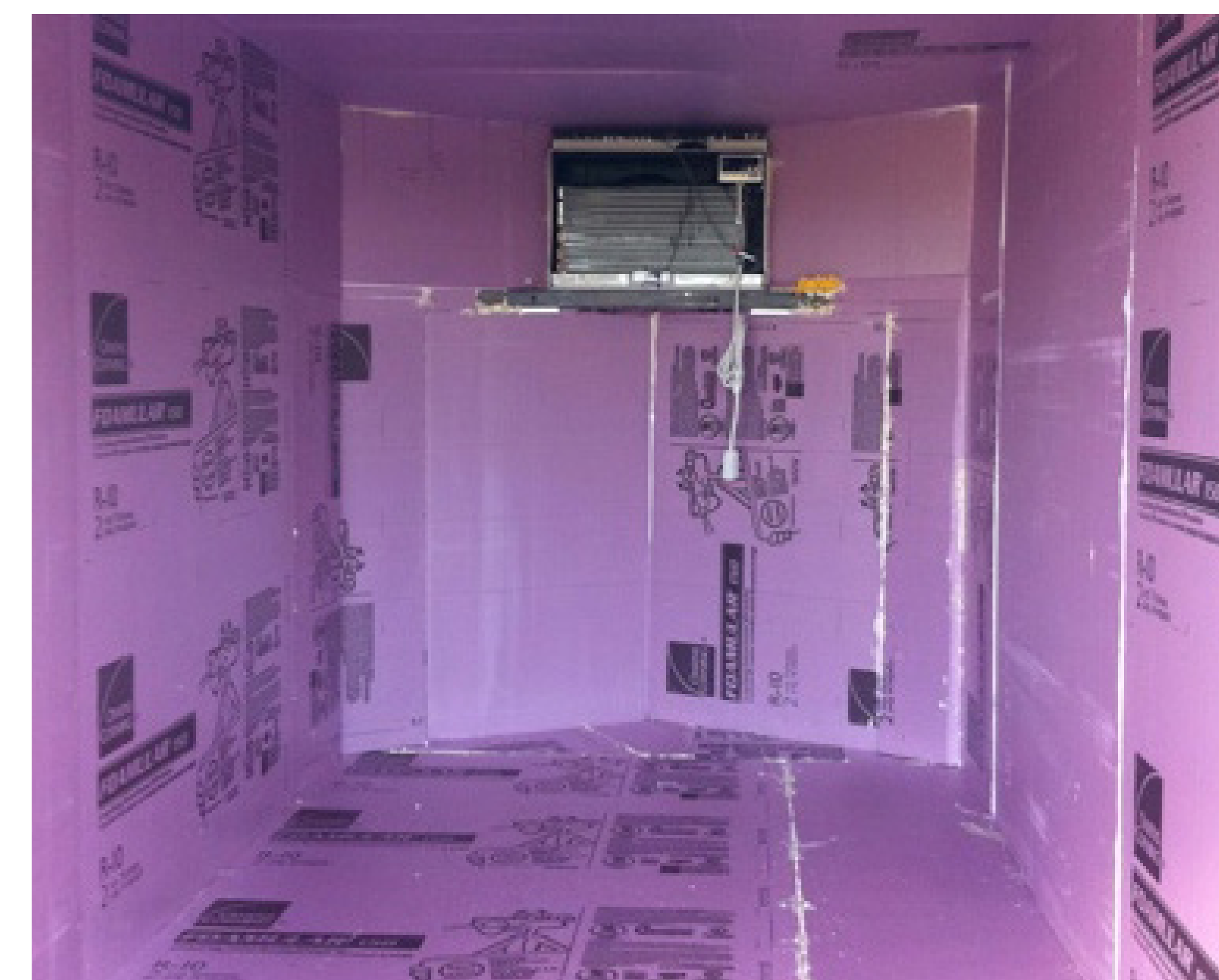
This insulating is funny business. We put four inches of foam board everywhere except the ceiling (because cold air sinks). The first layer went one way and then the second layer crossed over the first going the other way, in order to eliminate air gaps. (Photo: www.evergoodfarm.com/trailerbuild.html )
